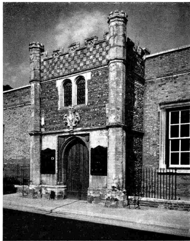
b. A recent view of the porch from the south-west.
