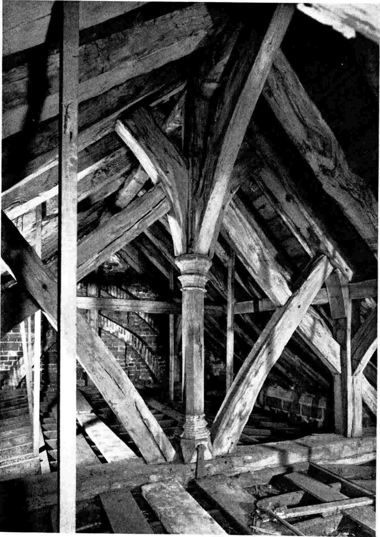
Truss at south end of hall.
